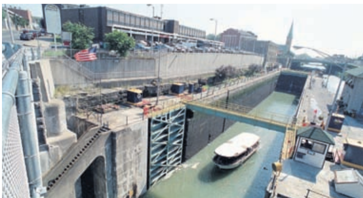
A boat moves through the double lock system on the Erie Canal in downtown Lockport, N.Y., Aug. 24, 1993.
